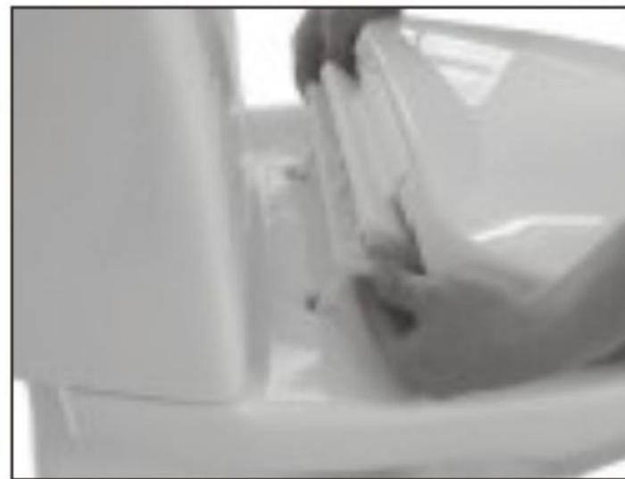
2. Position the seat cover on the toilet with bolt inserted into fixing hole
